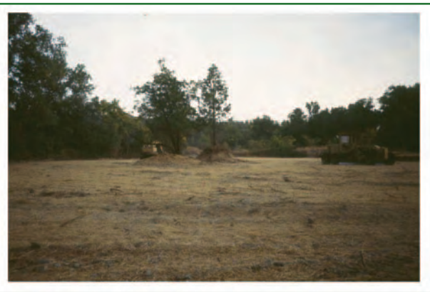
Above: Fill material was obtained from an upstream "borrow site" called Reading Bar, where the elevated floodplain was rarely inundated, which was then used to isolate a large salmon and steelhead stranding pit downstream. By removing the fill and leveling the site, Reading Bar has been lowered to an elevation that is more likely to receive floodwater under the controlled flow regime established by the dam. The trees at the center show the original grade of the site. Reading Bar has been restored with native riparian vegetation in a later phase of the project. • Source: Western Shasta RCD
