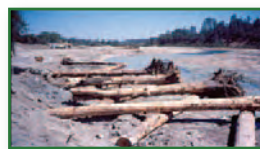
Above: The Western Shasta RCD redirected the Creek into the cobble-bedded channel that provides much better spawning habitat for fish.
