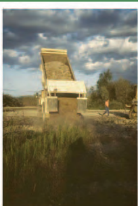
Above: Fill material was obtained from an upstream "borrow site" called Reading Bar, where the elevated floodplain was rarely inundated, which was then used to isolate a large salmon and steelhead stranding pit downstream. By removing the fill and leveling the site, Reading Bar has been lowered to an elevation that is more likely to receive floodwater under the controlled flow regime established by the dam. The trees at the center show the original grade of the site. Reading Bar has been restored with native riparian vegetation in a later phase of the project. • Source: Western Shasta RCD
