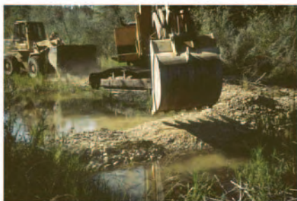
Below: Earthen berms were constructed to filter the water as it exited the plug area. Berms were also built across the high flow channel
